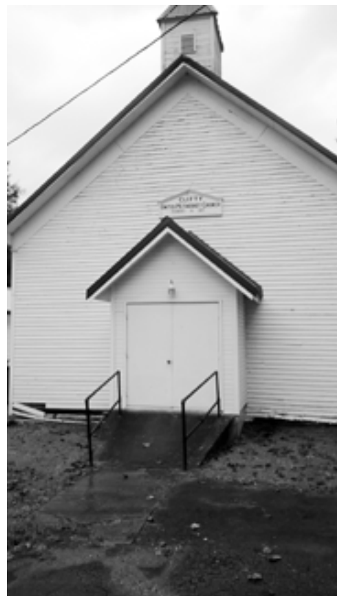
[7-KK] Entrance to Old Clifty Methodist Church where Rev. Cordy Pendergrass preached, founded 1891, now condemned due to age and damage
